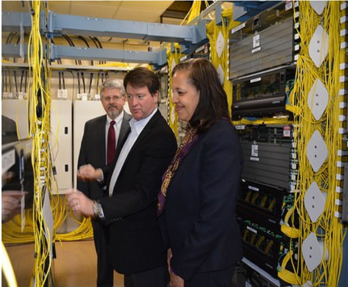
The Peoples Rural Telephone Cooperative recently completed their “fiber-to-the-premise” broadband project, providing access throughout two of Kentucky’s most economically distressed rural counties. In the image above, PRTC staff lead USDA Under Secretary Lisa Mensah on a tour of their operations center in McKee, Kentucky. Source: U.S. Department of Agriculture
